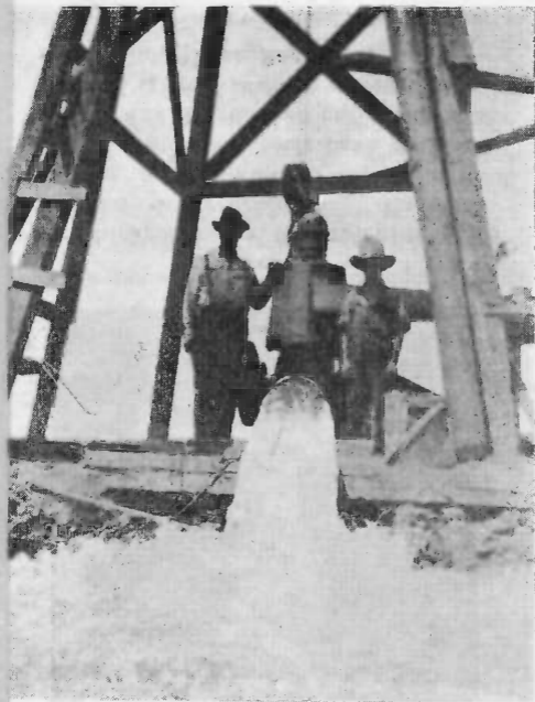
Pumping Plant of L. H. Sorey
