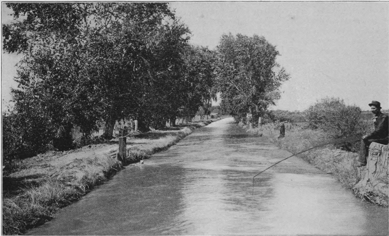
On the Grand Canal—Arizona Improvement Co.
