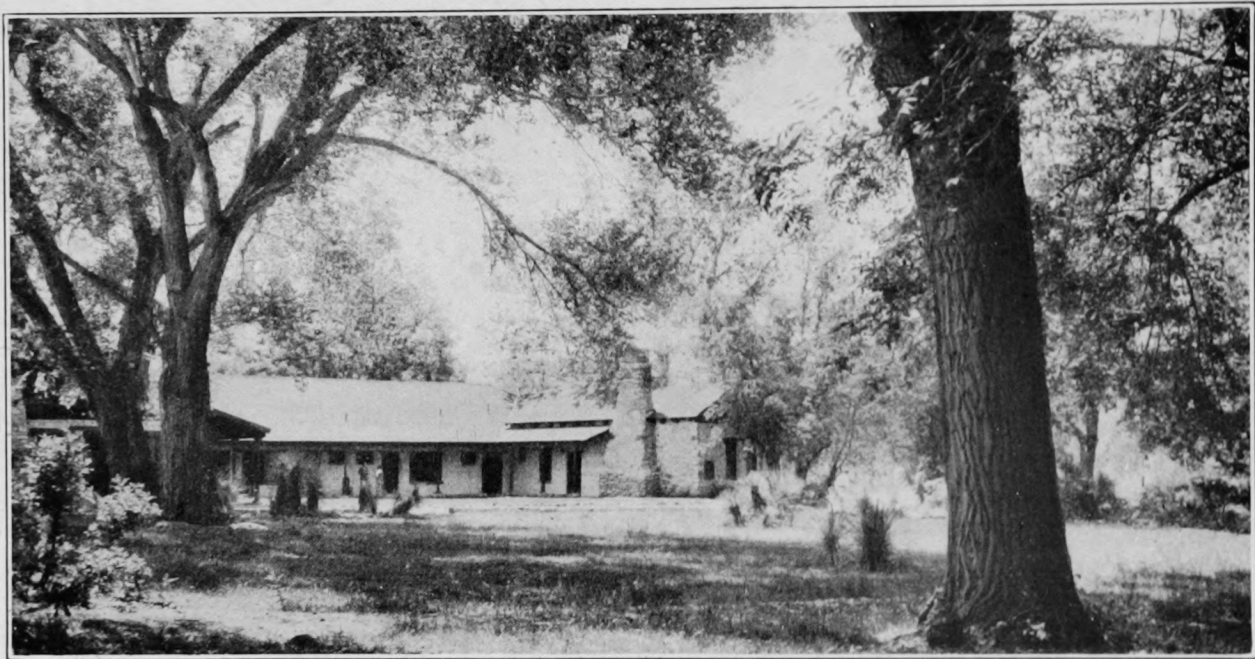
"The Soda Springs Ranch House Stands Amid Lovely Natural Surroundings"
