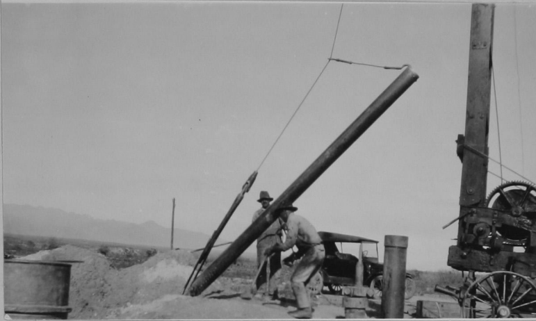
Fig. 17.- A method of emptying the mud-scow with only one line.
