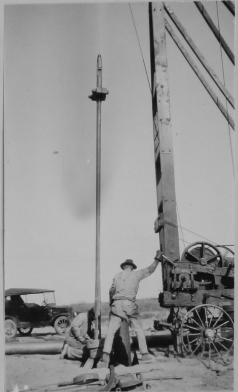
Fig.9.- A drilling stem with drive clamps bolted onto the upper wrench squares.
