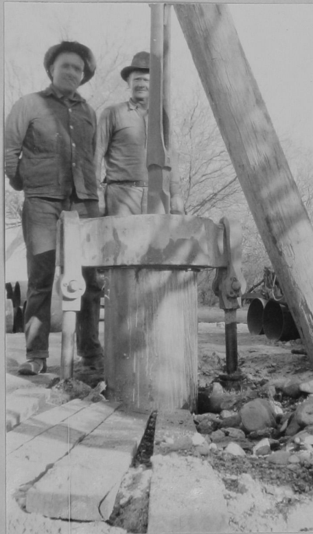
Fig. 18.- Forcing stovepipe casing down with hydraulic jacks.
