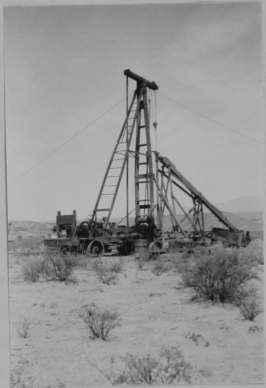
Fig. 5.- A large tractor rig of the California type. The frame work to the right of the rig was used in testing out the well with an airlift.
