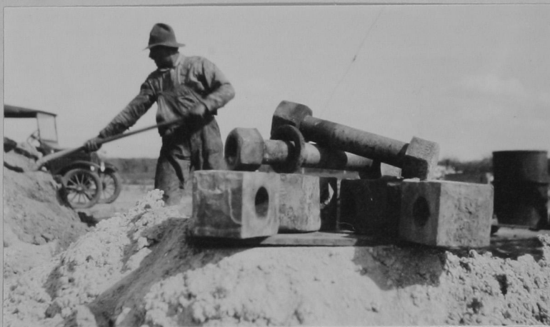
Fig. 15.- Set of drive clamps weighing about 150 pounds, used in driving casing.
