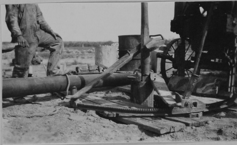
Fig. 13.- Setting up the tools with a circular track and jack.
