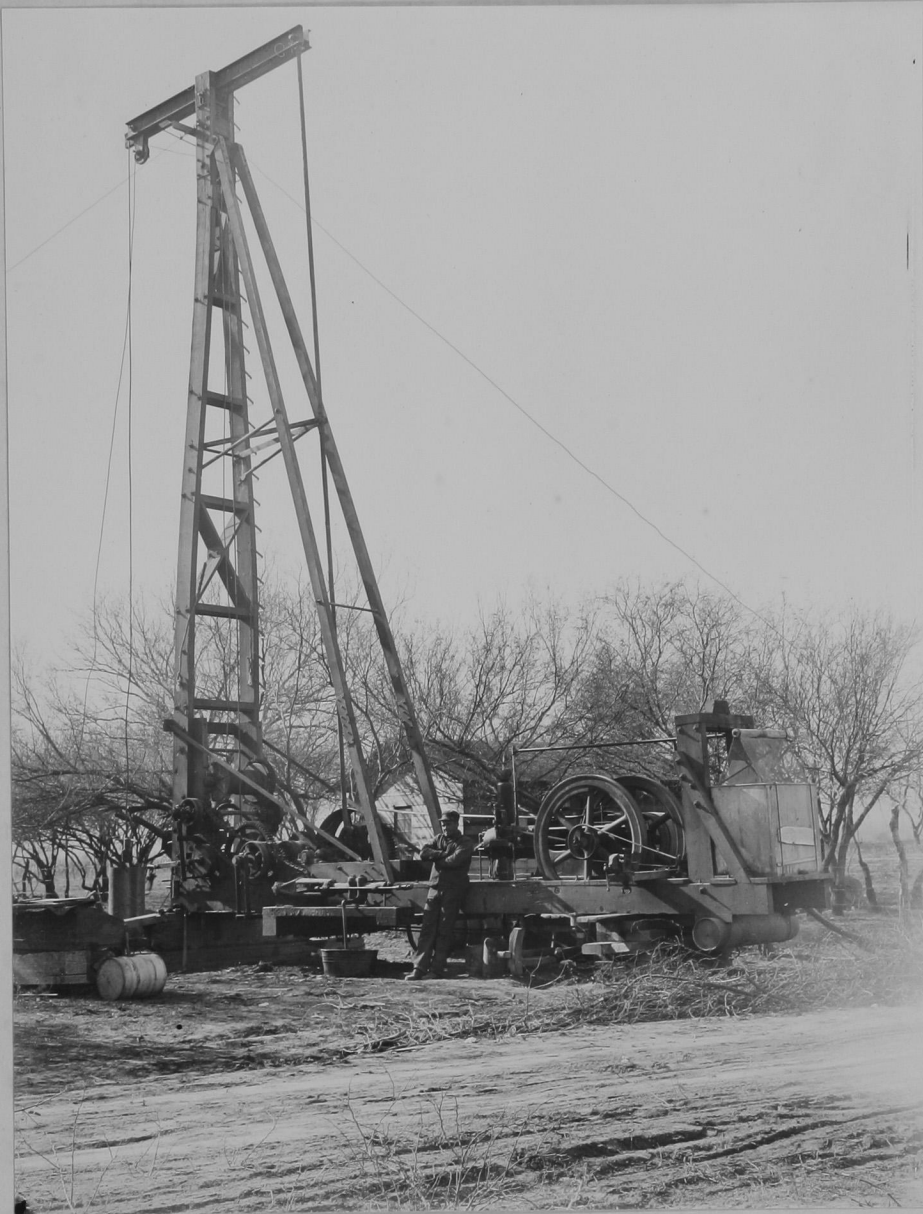
Fig. 3.- A California or mud-scow rig of the type most commonly seen in Arizona.
