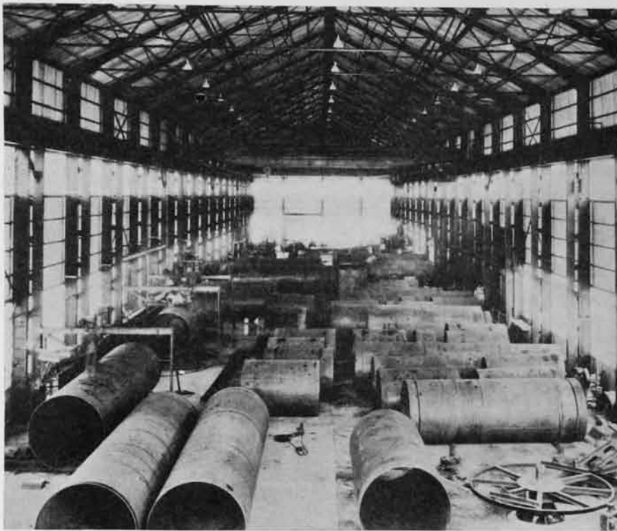
Fig. 2 (above)—Interior of shop during fabrication of 8½-ft. pipe sections, first to be built. View is toward receiving end of plant, with welding machines at left.
