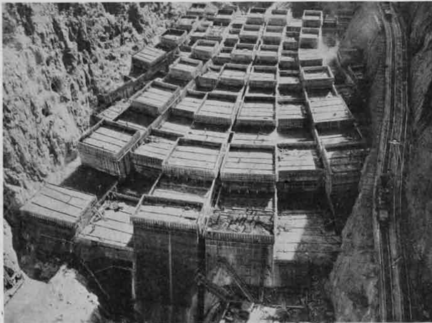
Fig. 1—Early progress on a 3,400,000-cu.yd. mass of concrete, 650 ft. thick from up- to downstream face, that presented a great many problems of unprecedented magnitude. Note the columnar construction, the central 8-ft. slot for the cooler-pipe headers and concrete placing under way on one of the blocks in the foreground.
