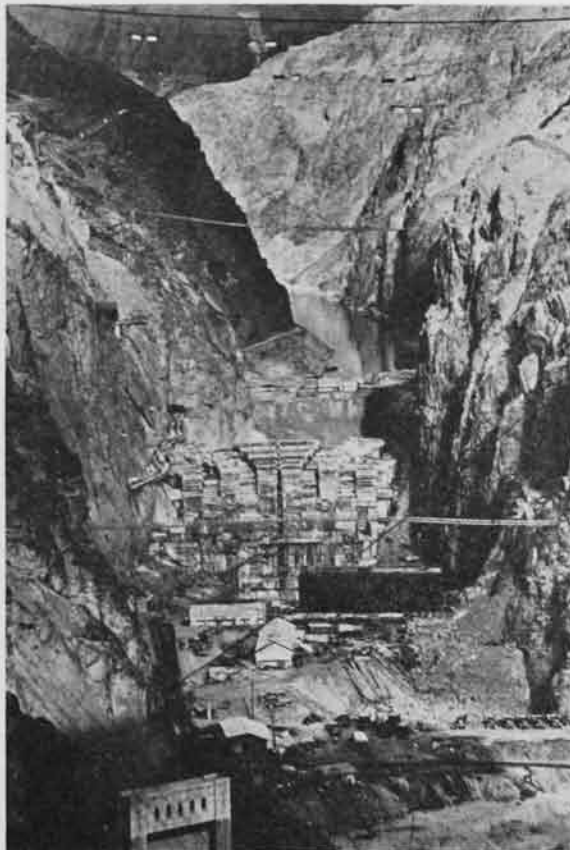
Black Canyon as it appears at present. Nearly 1,000,000 yd. of concrete have been placed in Boulder Dam.
