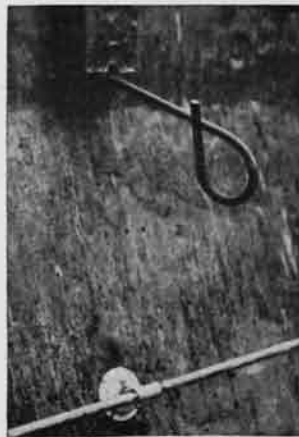
Fig. 5—Details of forms fastenings: Cooling pipes are laid on the surface (left) immediately before the lift is placed. She-bolts and hooked rods (center) embedded in the top of the lift provide for holding the cantilever forms for the next lift. Outlets for the grout system are nailed to the forms. Note the keyways produced by the forms.
