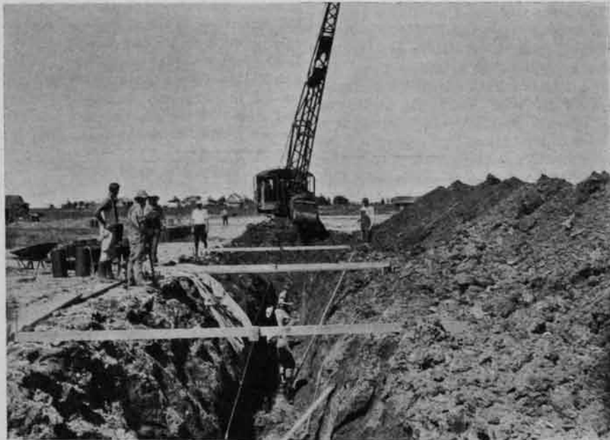
Construction of Newell town-site drain, Belle Fourche project, South Dakota
