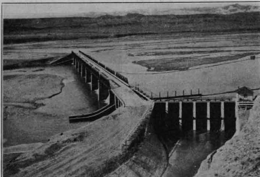
The Wind River diversion dam on the Riverton project, Wyo.
