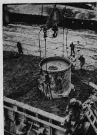
Fig. 6—Concrete buckets are brought to rest on the surface of the lift (left), which releases the safety catches, and the take-up is then made with the lines attached to the rim, which has an action of lifting the bucket off the concrete (right). Note the consistency and the details of the forms.
